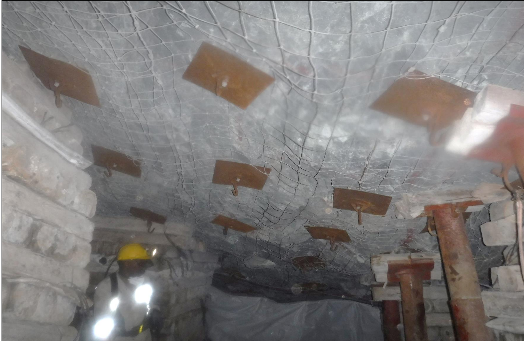
Supported with Steel nets, Hydrabolts and 300mm x 300mm plates
