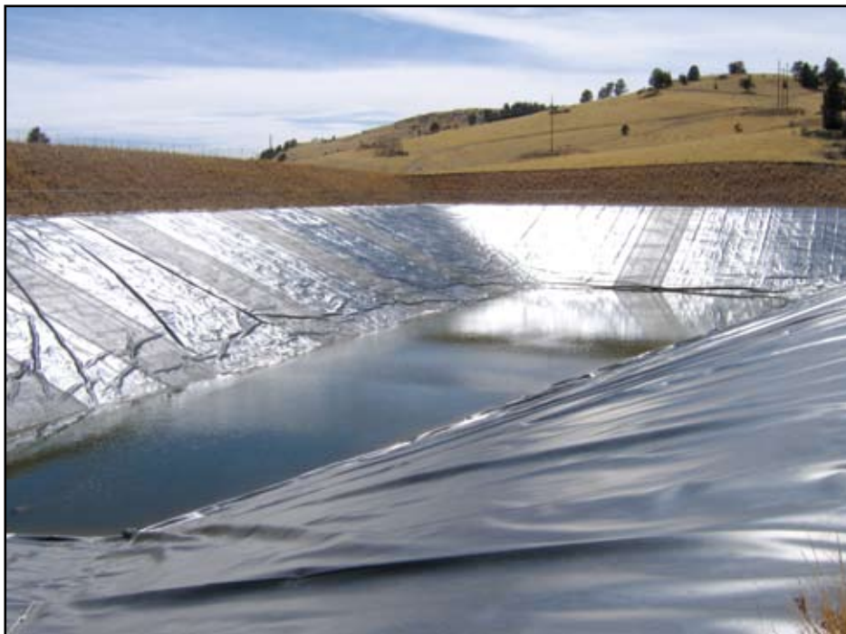
Figure 6-14: Example of a lined water storage facility
