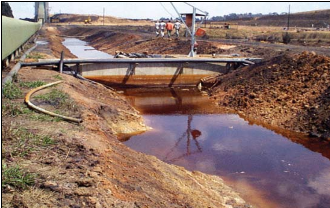
Figure 6-8: Groundwater seepage cutoff trench
