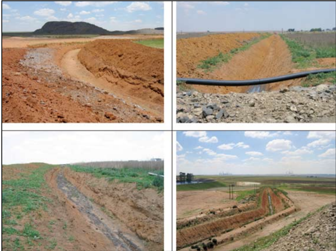
Figure 6-4: Examples of water separation trenches and canals
