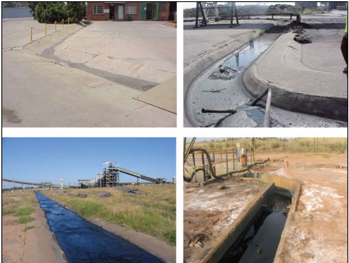
Figure 6-11: Examples of lined conveyance structures
