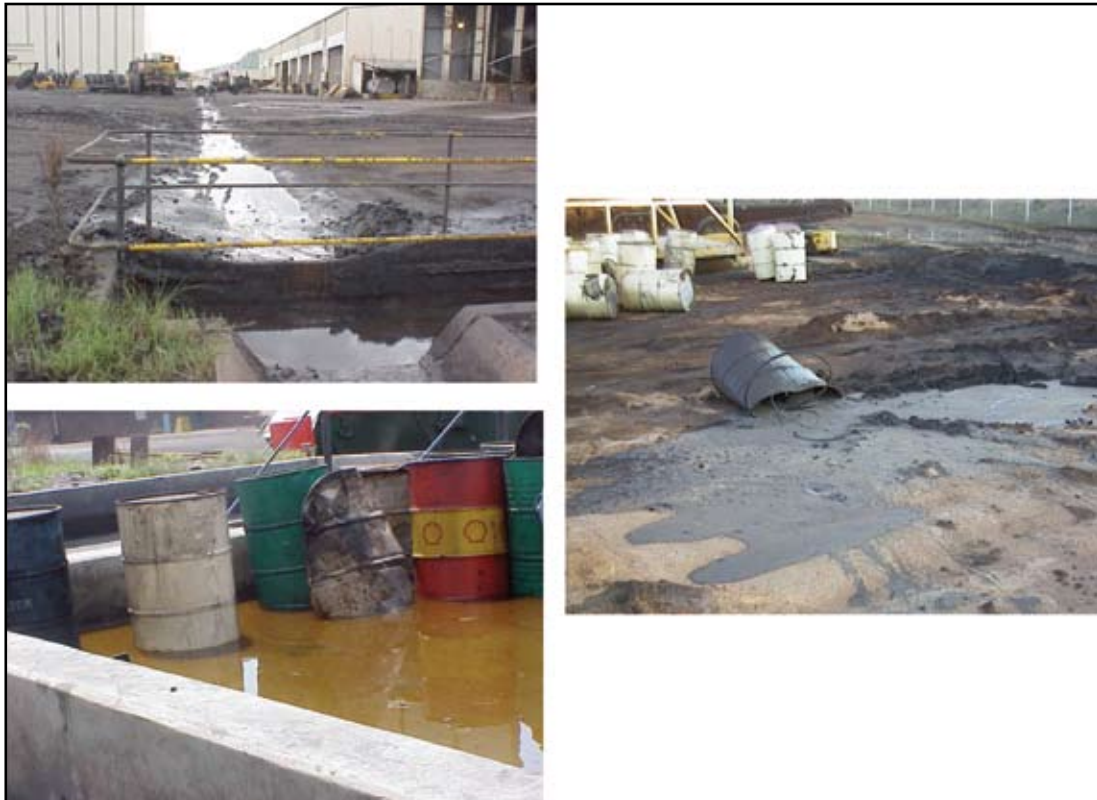
Figure 6-22: Examples of poor practice for silt traps and maintenance areas
