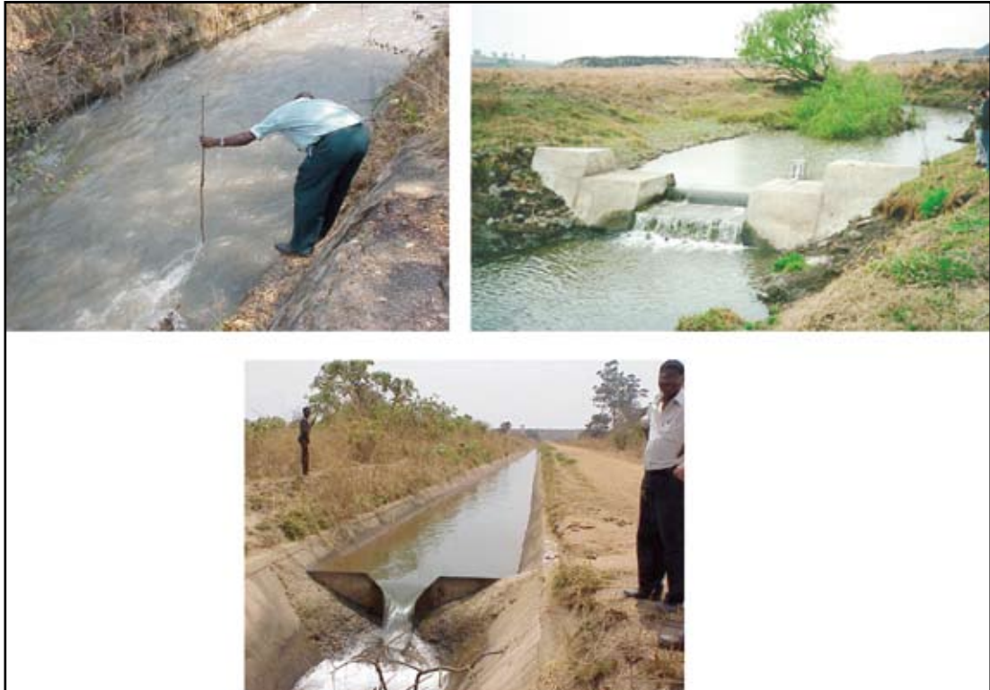
Figure 6-28: Monitoring flow in surface water channels
