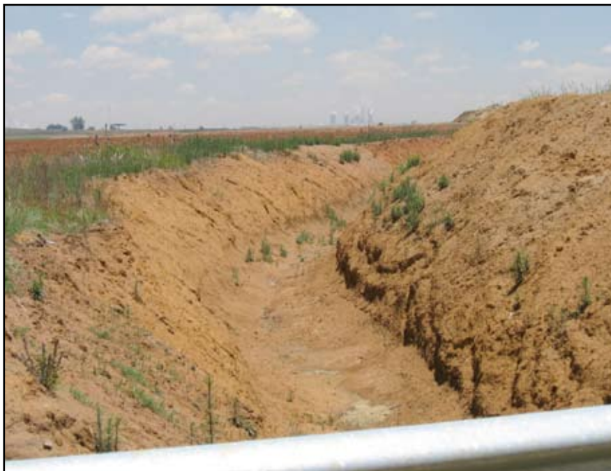
Figure 6-3: Illustration of a clean water cutoff canal
