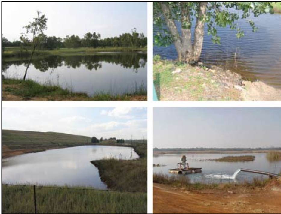
Figure 6-13: Examples of water storage facilities
