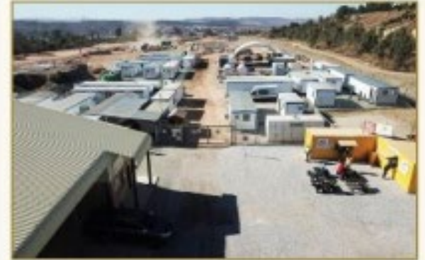
First gold — build-out around a working mine.
