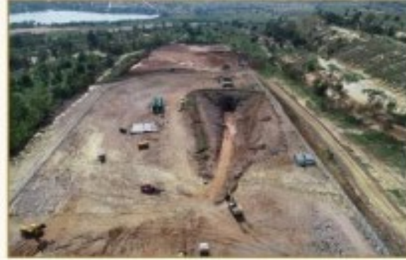
Breaking ground — the box cut carved into cleared earth.
