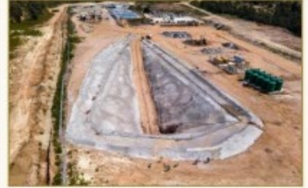
Box cut collared and shotcreted; the decline portal established.
