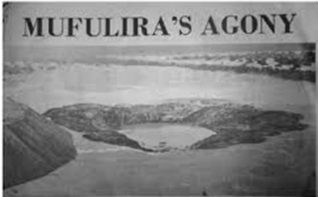
Figure 1: Aerial view of the sinkhole at Mufulira No. 3 Dam (Source: Times of Zambia, 24 October 1970.)
