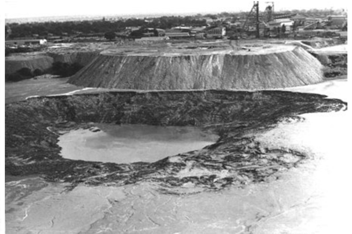
Figure 1: Aerial view of the sinkhole at Mufulira No. 3 Dam (Source: Times of Zambia, 24 October 1970.)
